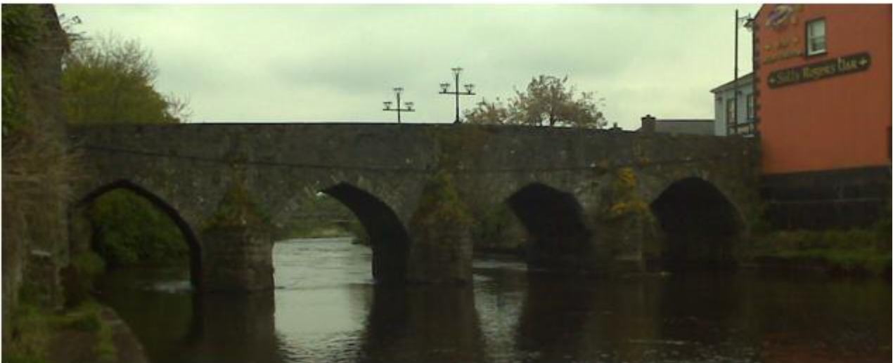
Figure 5-2 - R161 Old bridge - Blockage Test (CFRAM Survey)
